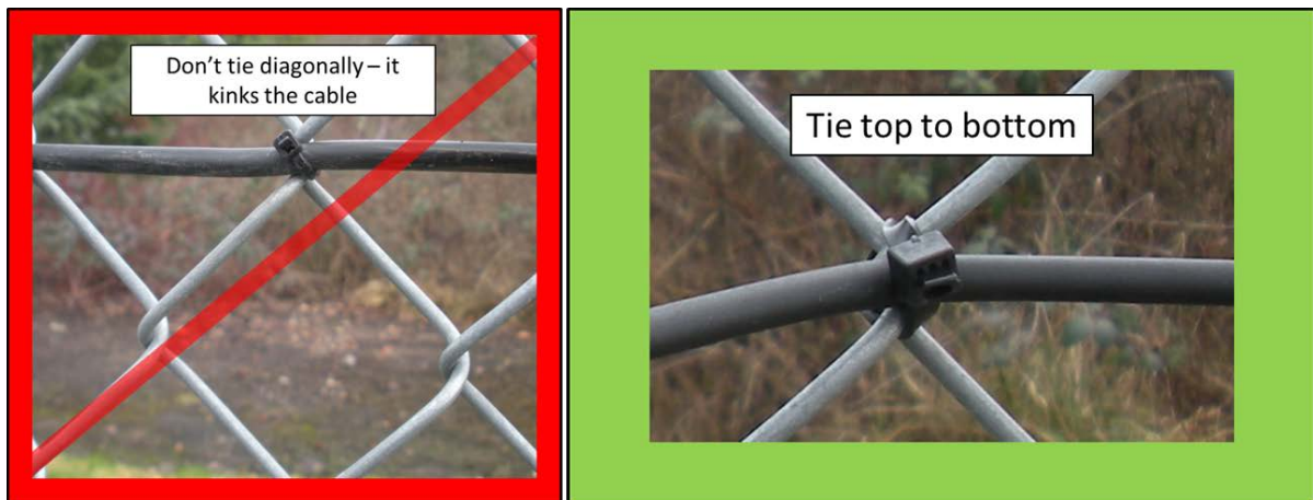
Figure 2-3. Loop the zip tie vertically to avoid kinking the cable.
