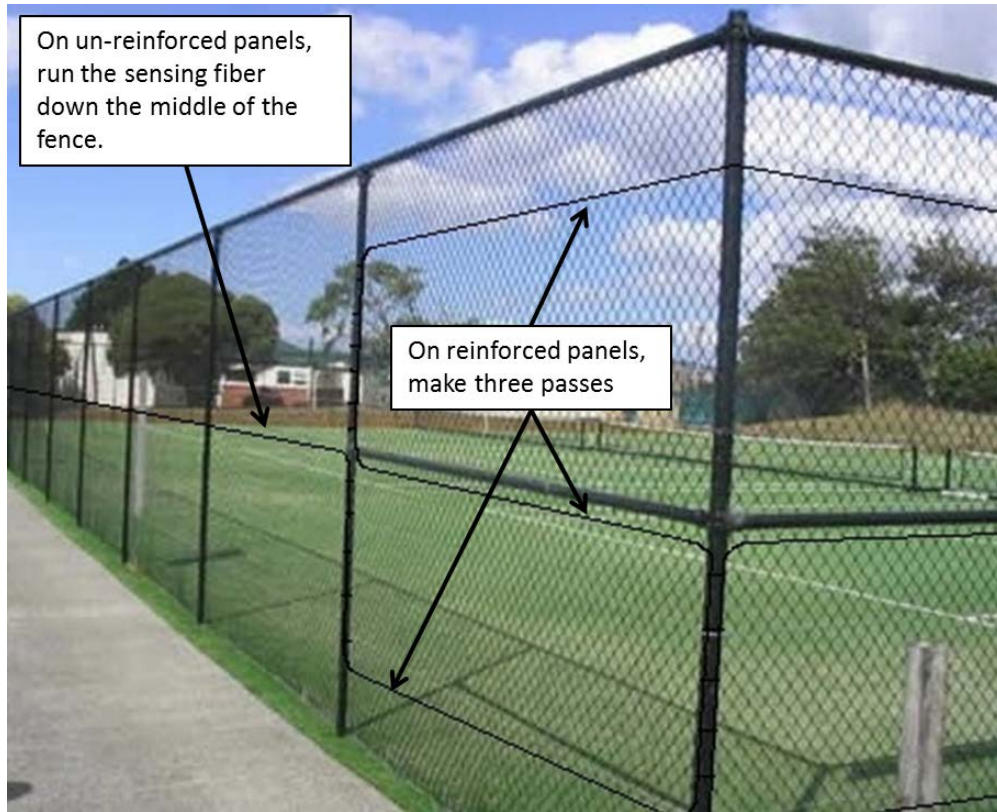
Figure 2-5. A single run of cable is sufficient for non-reinforced panels, but three passes of cable may be necessary for reinforced sections.
