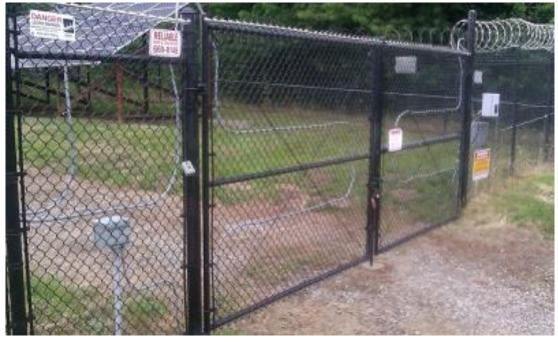
Figure 6: Gate Protection with Fiber–Optic Sensor
