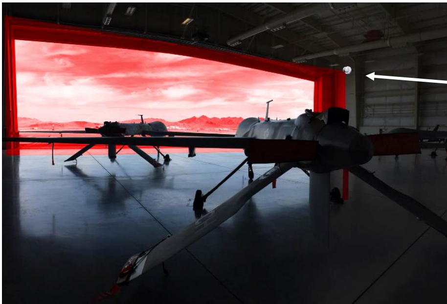
Figure 4: Vertical mount hangar door protection
