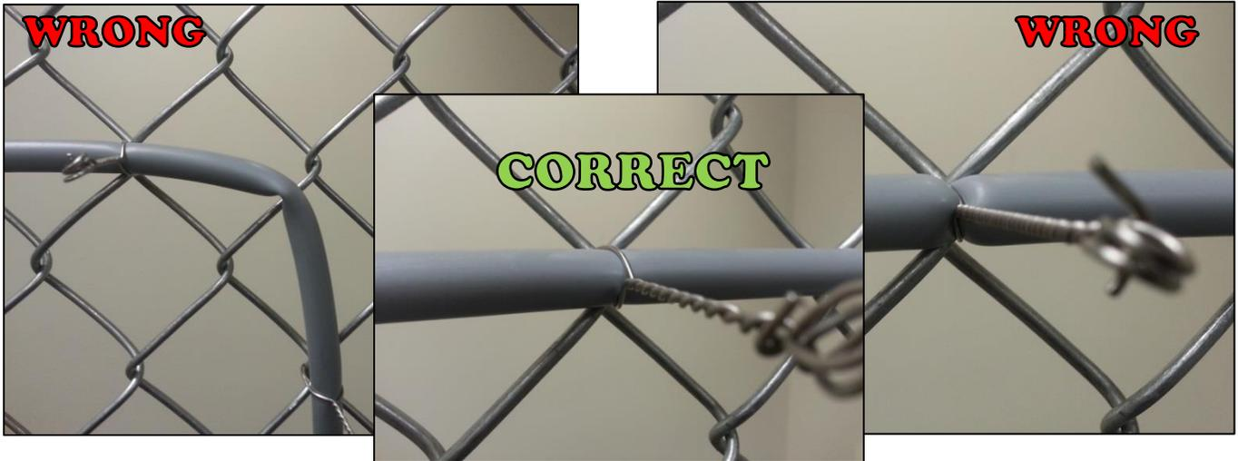
9. Fence fabric should be in good repair; deflection  $\leq 2''$  @ 30lbs for commercial grade fence or 50lbs for military grade fence; Repair loose sections; Tighten loose signs that are attached to the fence; Clear brush, trees or other obstructions that could cause nuisance alarms.
