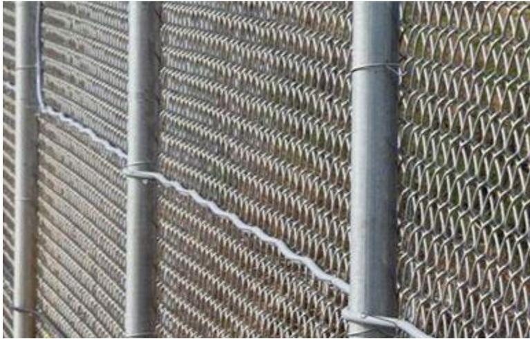
6. Conduit should be affixed to the protected side of the media material while applying approximately 30lbs of tension. This will help to eliminate sagging of sensor during hot and cold weather cycles.
