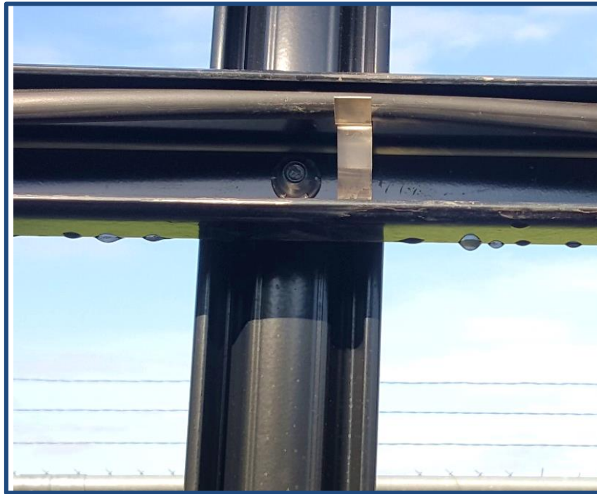
Figure 5: Sensor Wire Clips (SWC100) Securing SC-4 and SC3-C
